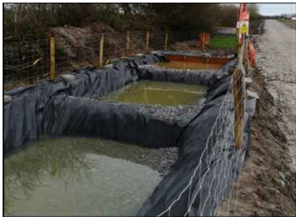
Completed Settling Pond System
